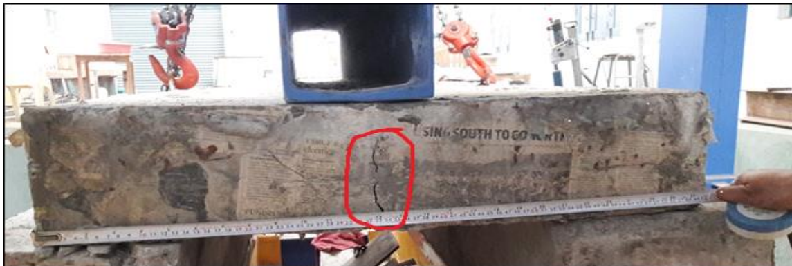
Figure 7: Cracks in bubble deck slab
