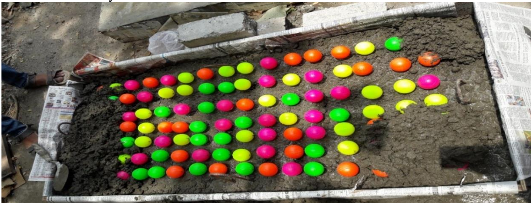
Figure 2. Slab with Bubbles
